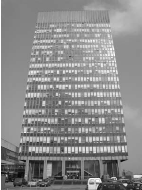
Figure 9.2 The same building
